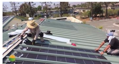
Figure 3.1. In-roof mounting BIPV system (top)
