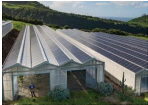
Figure 5.4. PV greenhouse (Source: Akuo)
