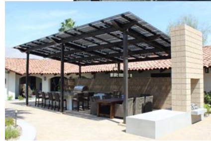
Figure 4.5. Solar carport (top) Solar canopy (bottom)
