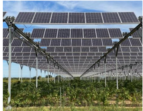
Figure 5.3. Elevated PV with tracking (Source: Sun’agri, REMTEC)
