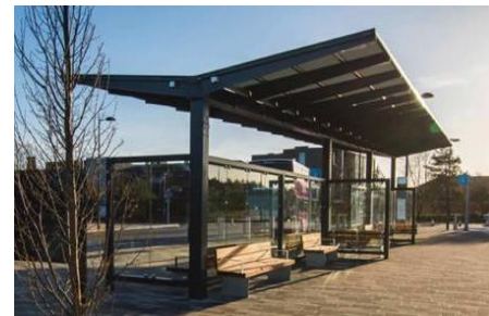
Figure 4.6. Example of IPV bus shelters
