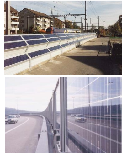
Figure 4.1. Cassettes PVNB along railway (top) Bifacial vertical PVNB along highway (bottom)
