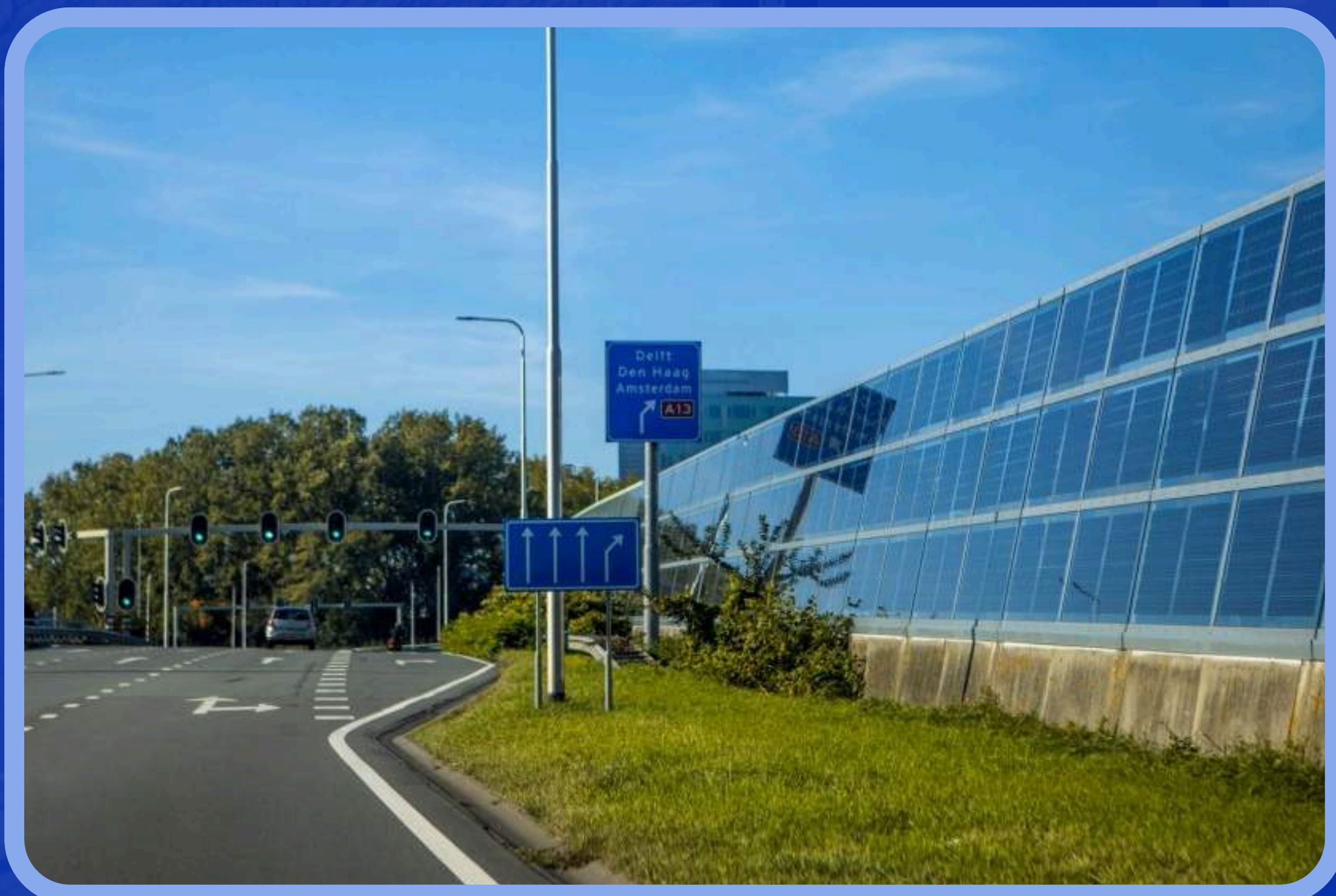
A PVNB installation in the Netherlands
