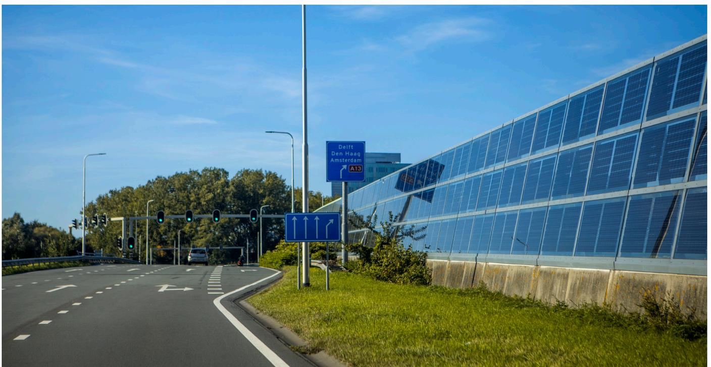
Since the main functionality of a noise barrier is providing noise abatement, new PVNB products will therefore have to fulfil the dual role of noise abatement and energy generation in a single integrated element. Based on this notion, SEAMLESS-PV project is developing new PVNBs, that still focus on acoustic attenuation (in compliance with regulation's standards and requirements) while efficiently producing renewable energy at a cost-competitive price.
