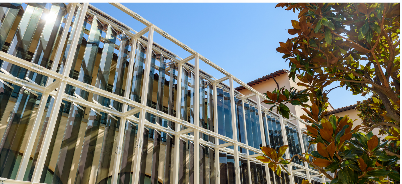
Solar panels integrated in the facade of a University building in Florence.
